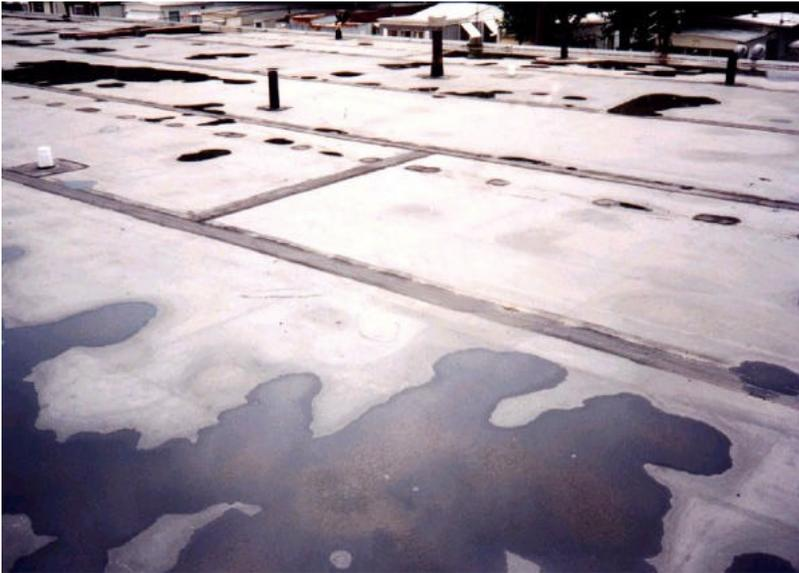
*This aged EPDM roof has been repaired with newer membrane – notice the light gray reflective color of the aged membrane.*
